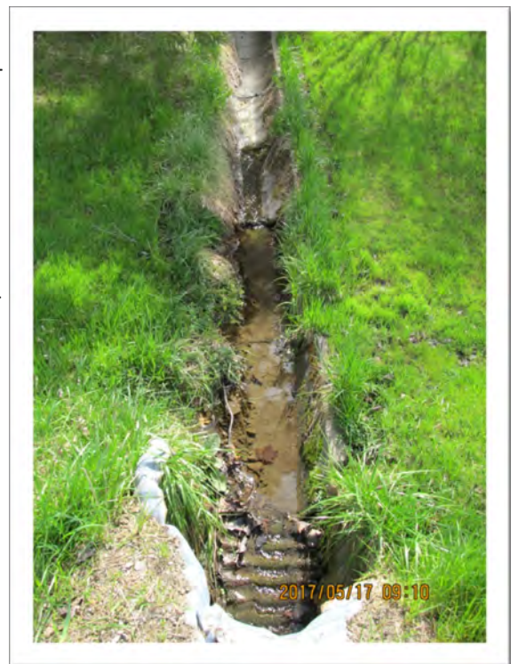
Figure 5. Stream channel straightened and confined via concrete drainage half pipe resulting in loss of habitat.
